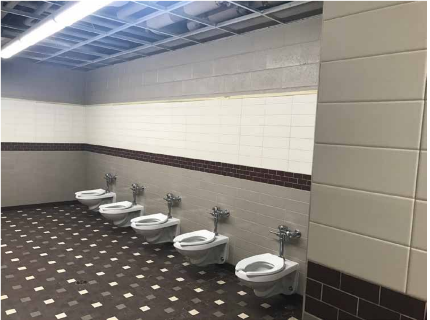
New Restrooms getting prepared for partitions
